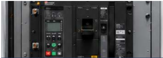
DRAW-OUT BREAKER Easy maintenance with draw-out design for faster inspection and replacement
